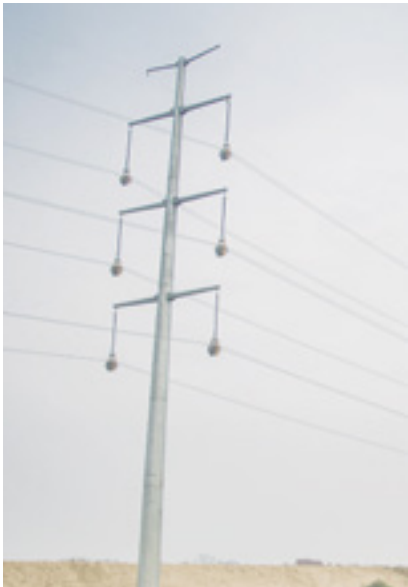
400kV Monopole Project at Noida for UPPTCL
