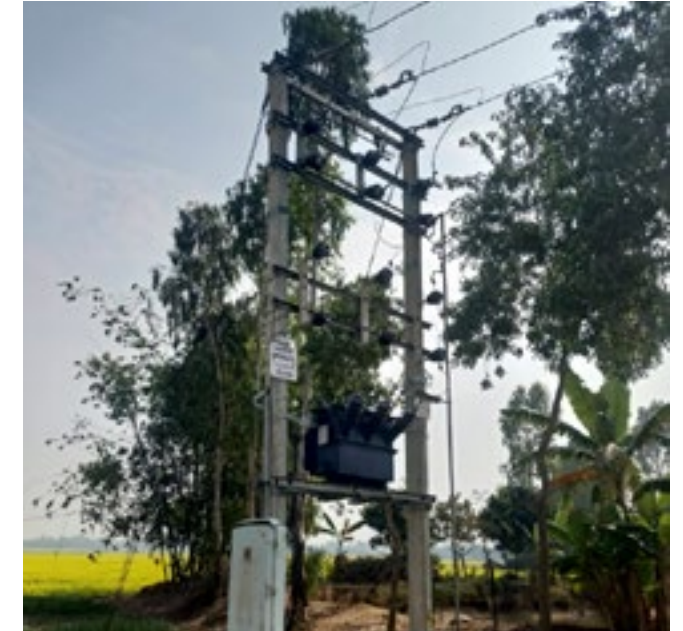
Feeder Separation Projects
