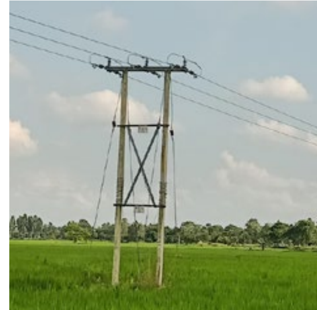
Rural Electrification Works
