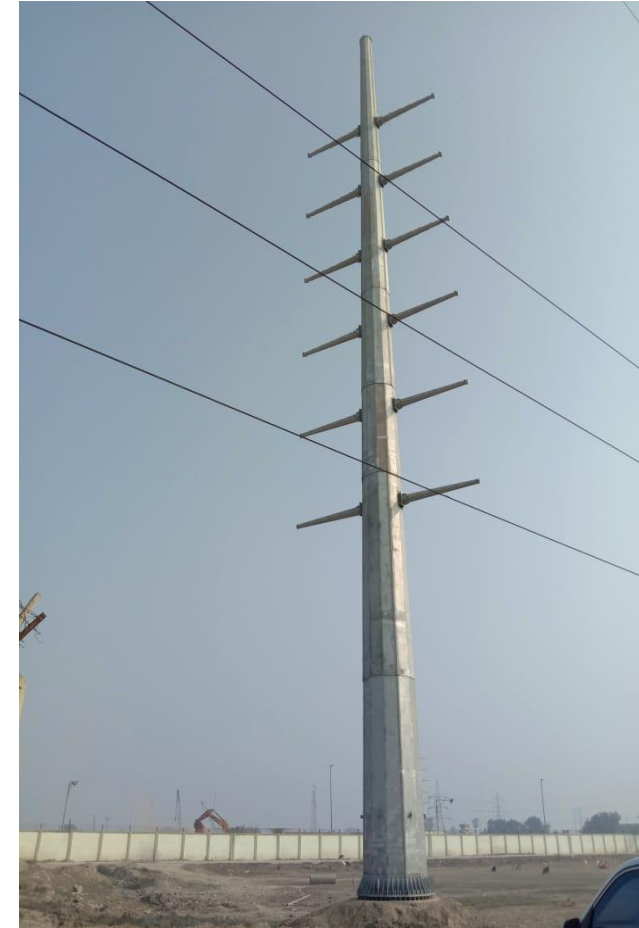
First 220 kV multi-circuit Monopole, Bihar State Power Transmission Company Limited
