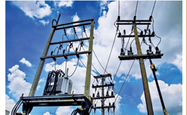
Feeder Separation Projects
