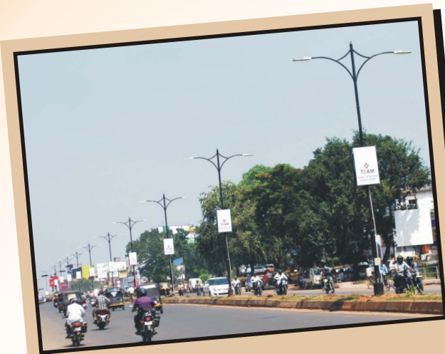
POLE POSITION: INSTALLATION OF ROTHAY POLES IN BHUBANESWAR
