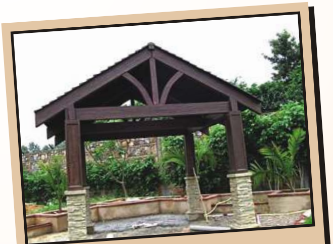
COUNTRYSIDE CREATIVITY: GFRP LODGE INSTALLED AT A FARMHOUSE IN CHATTARPUR, NEW DELHI.
