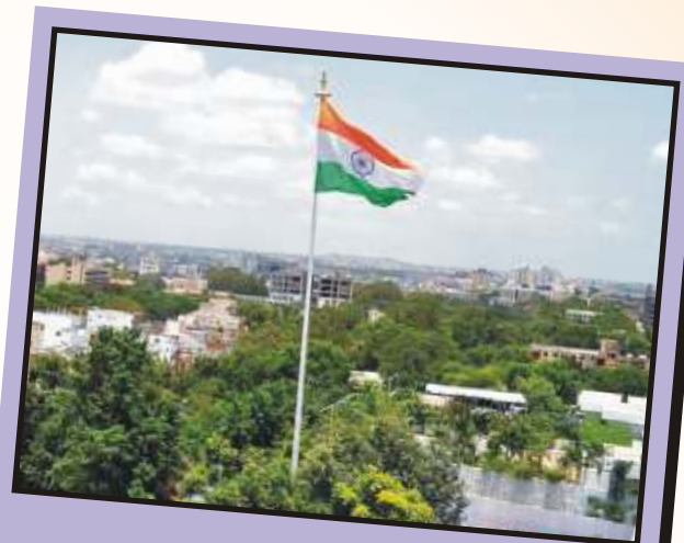
HIGH AND MIGHTY: 30.5 Mtr FLAG MAST INSTALLED ON ROAD NO. I, BANJARA HILLS, HYDERABAD.
